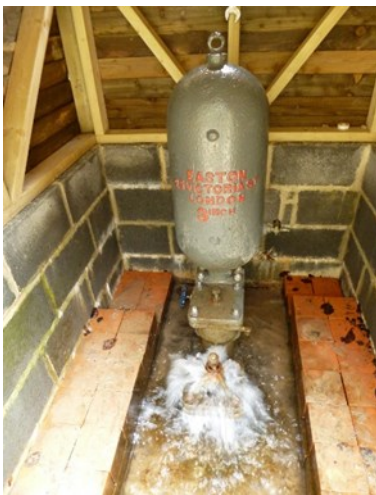
Figure 1: Traditional ram pump
